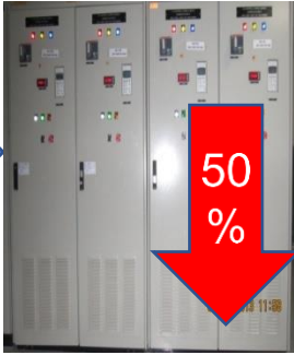
After: Installed 22 No's VFD s for all the bag filter fans
