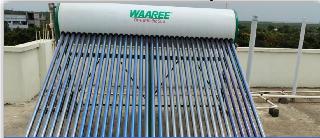
Solar Water Heaters for Colony – 150 Flats
