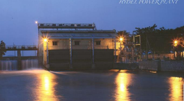
HYDEL POWER PLANT, NEKARIKALLU – 8.25 MW
