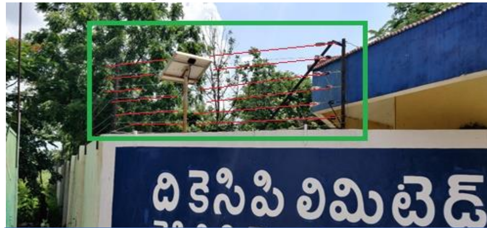
Solar Fencing around the Residential Colony
