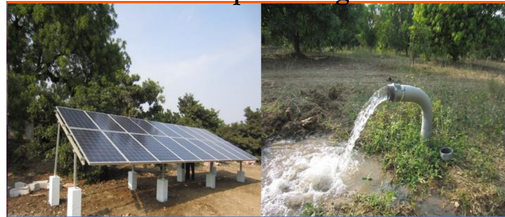
Solar Water Pump at Mango Garden
